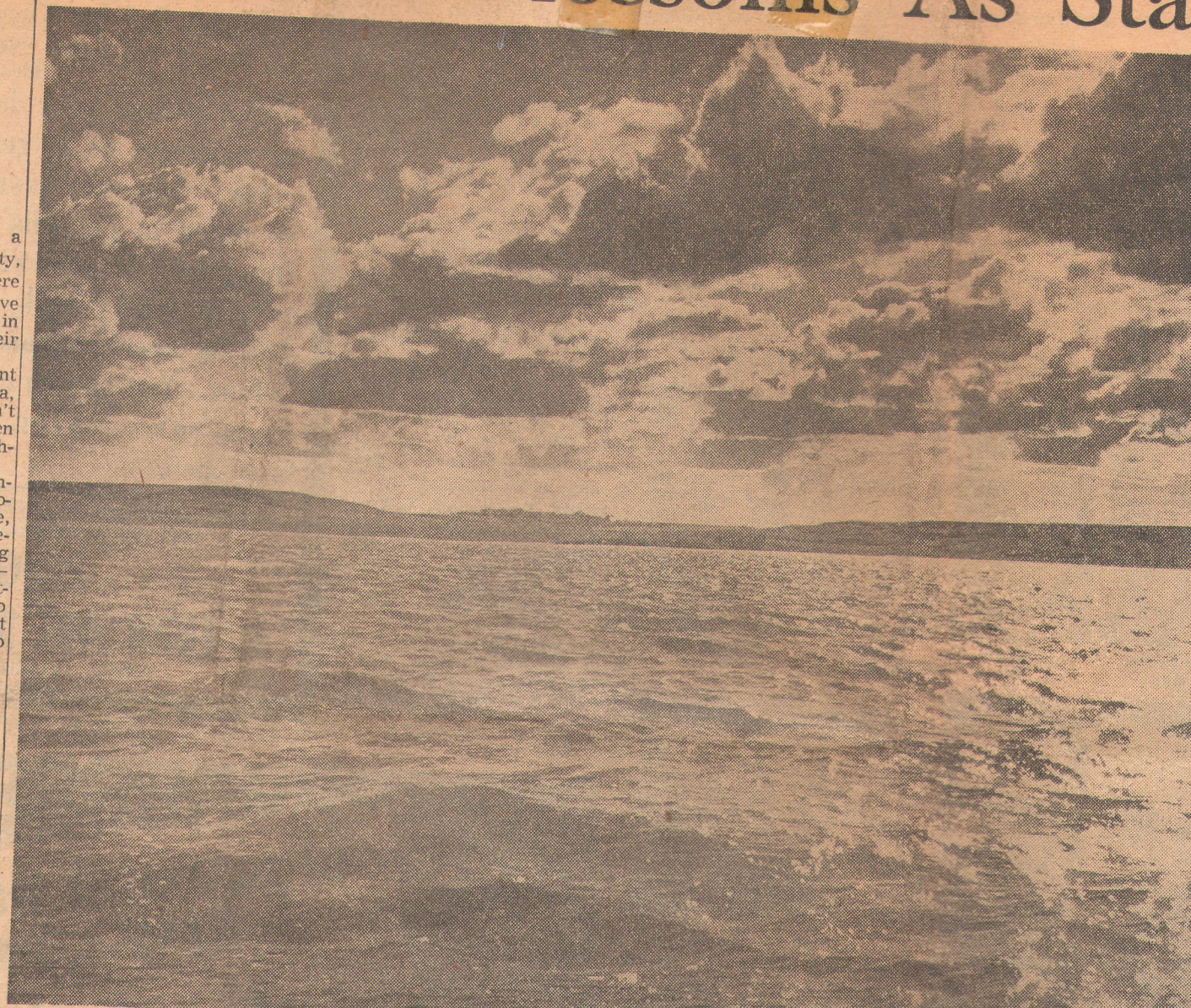
LOOKING ACROSS Lake Ashtabula, this picture shows the average width of the Baldhill Dam reservoir, which extends about 35 miles north of the dam. The shoreline ranges from gentle slopes
